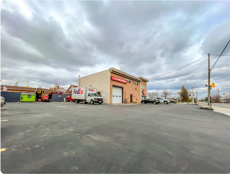
Fig. 8.2 The vehicle plane at ground level, from the rear lot looking north, April 2025. The courier truck is parked against the blank south wall. This is the plane a walking customer must cross.
